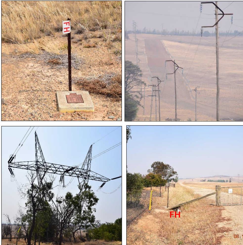
Figure 10 – Photos of existing infrastructure
